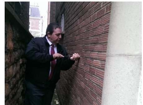
Installer checking feasibility of cavity wall insulation
