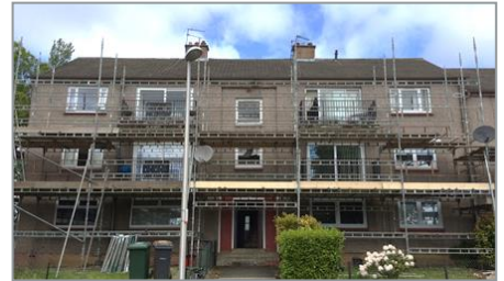
Case study block during retrofit
