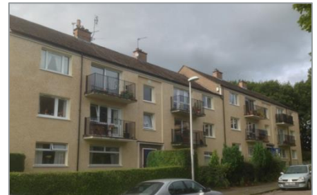
Case study block post retrofit
